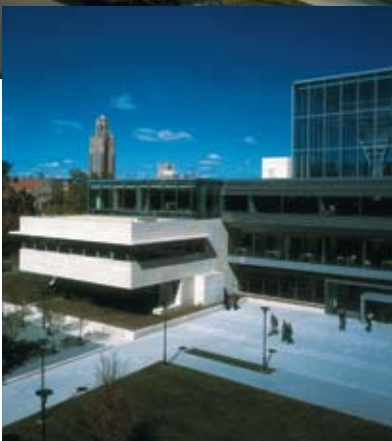
The Charles M. Harper Center at the University of Chicago's Graduate School of Business features thinly cut limestone cast into precast concrete panels to achieve the look of masonry with additional benefits.
